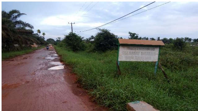
Figure 4: Poor Main Road
